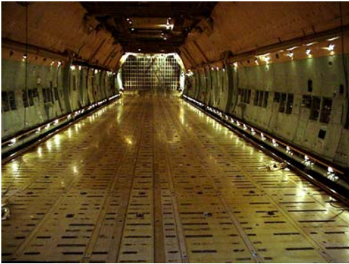
Thermal and acoustical sidewall panels installed in cargo area.
